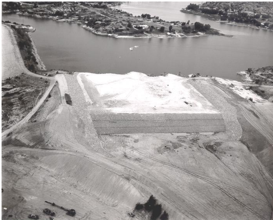
Lake Tanglewood Dam emergency spillway on August 1, 1977 after construction of erosion control improvements.
