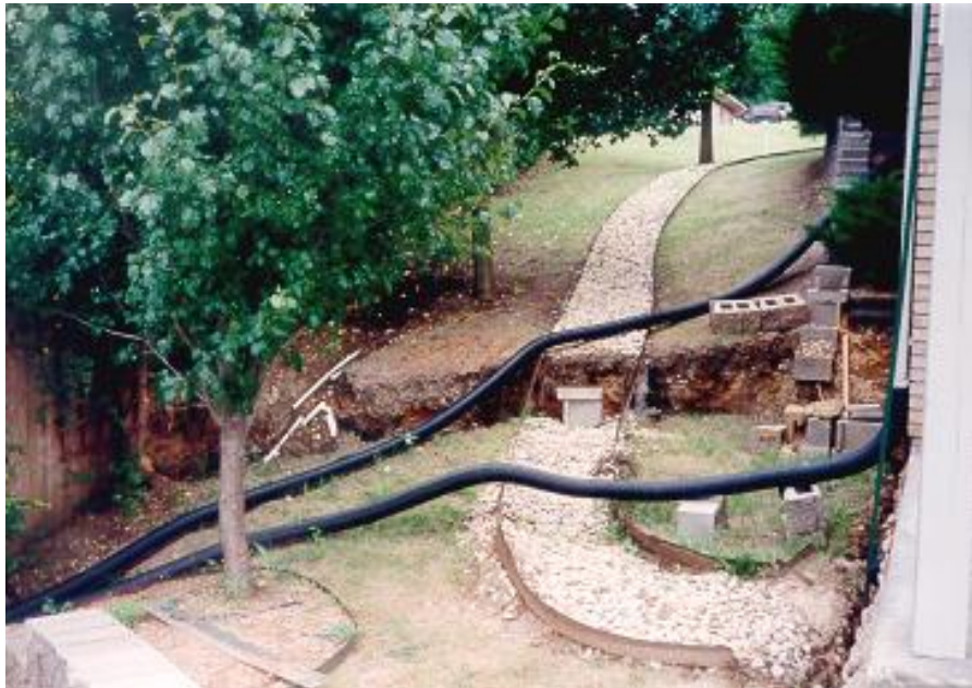
Separated scarp of landslide extending under home in Dallas area.
