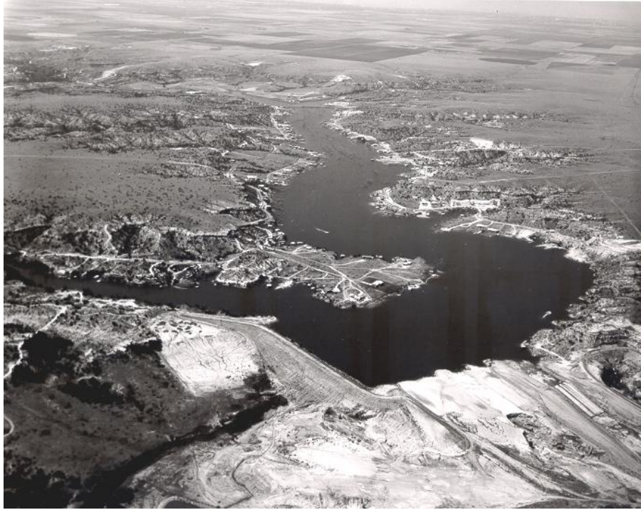
Lake Tanglewood Dam emergency spillway on June 30, 1966, prior to construction of erosion control improvements.
