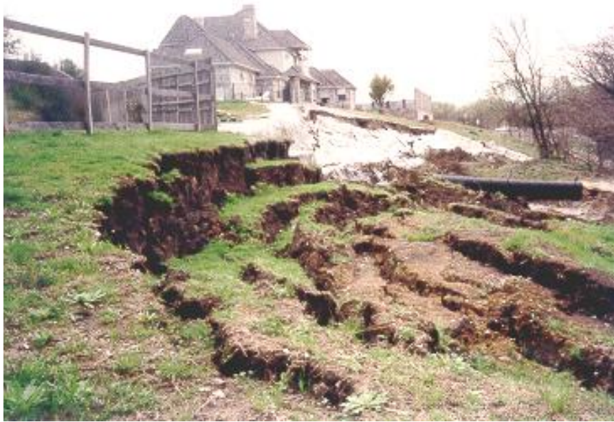
Failed attempted control of landslide using shotcrete next to homes. Note the shotcrete failed as slide continued to move.
