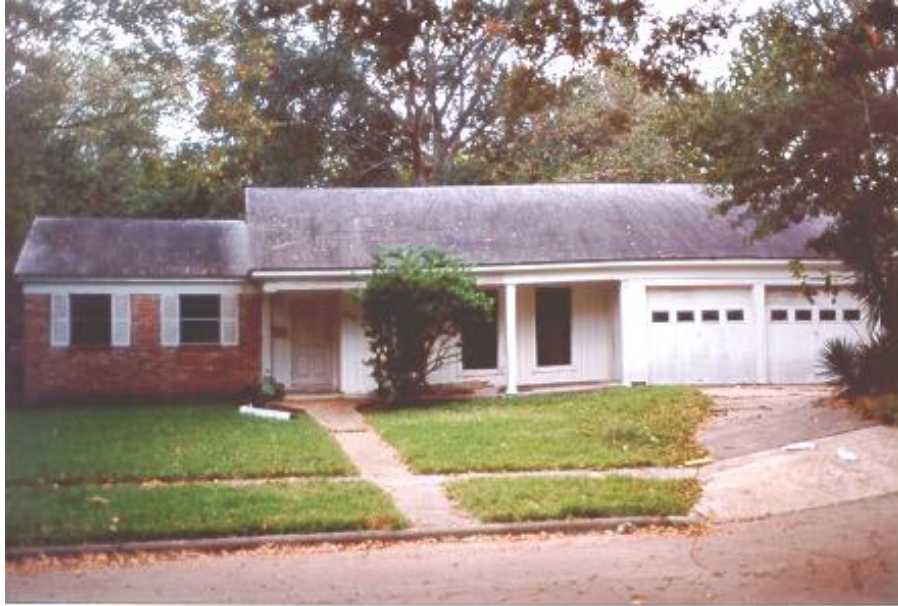
Fault extending under home at 1307 Moorhead in Houston. Note the downthrown block is to the left. The home is settling to the left with fault movement.
