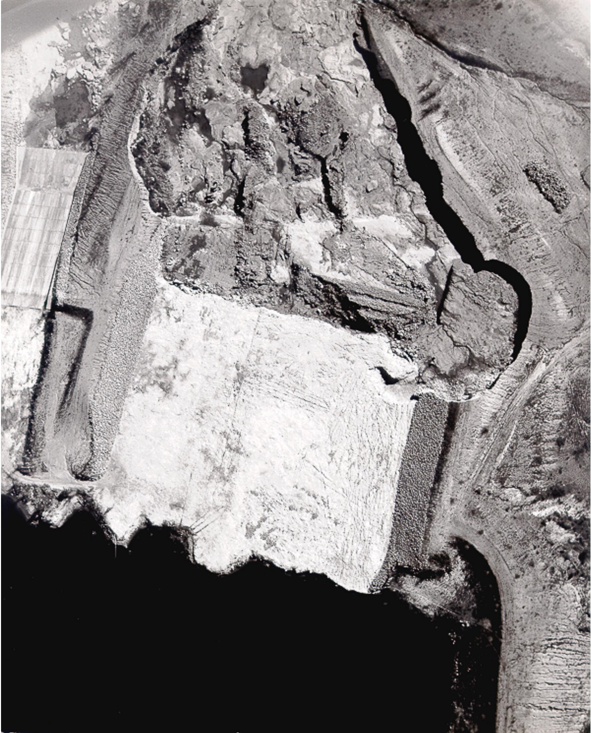
Lake Tanglewood Dam emergency spillway following May 27, 28, 1978 rainstorm that resulted in flow over spillway. Note failure of the erosion control improvements and significant downstream erosion.
