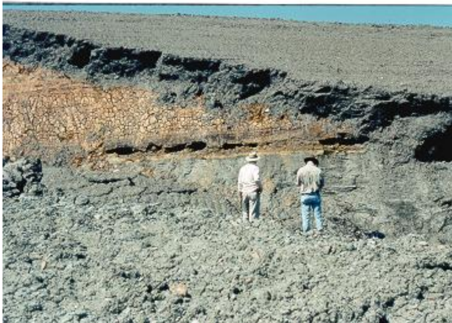
Geologists standing on slide block of failed western wall looking across block separation at landfill scarp.
