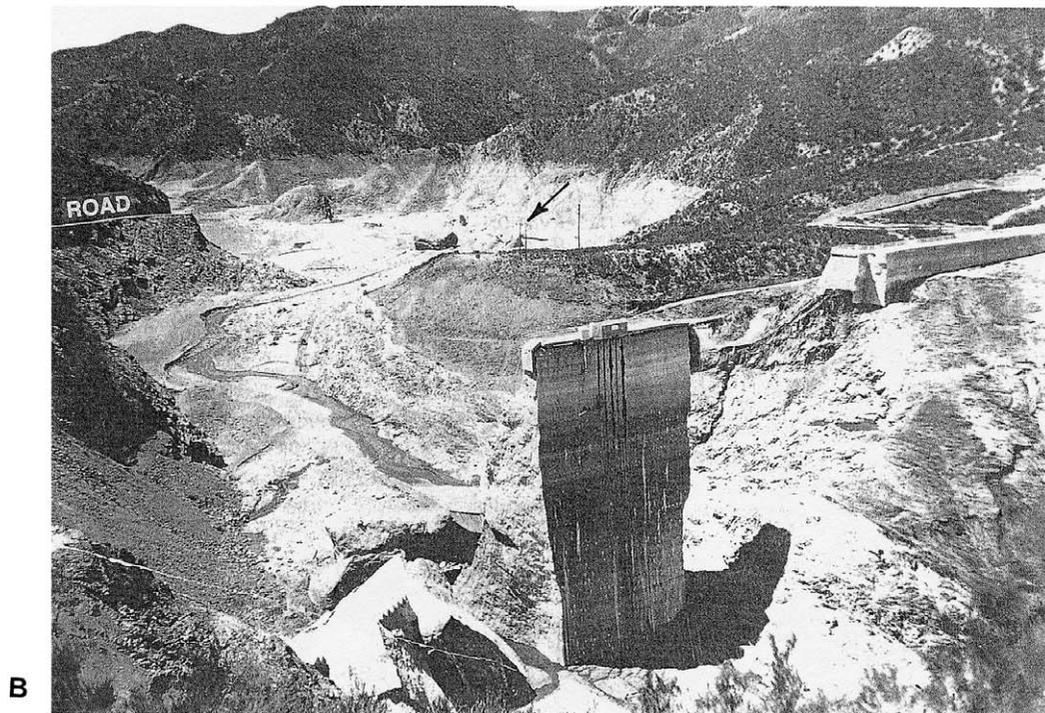
Figure 22. (A) St. Francis Dam as viewed from the north, as it appeared just after its completion in May 1926. The dam was 200 ft (61 m) high and is situated on a fault that separates sandstone from schist. (B) St. Francis Dam, viewed from the north, after the collapse and resulting flood. (Photos courtesy of Ventura County Museum of History and Art.)
