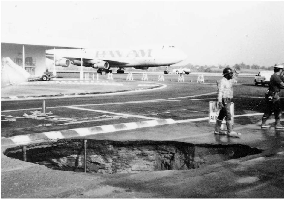
Figure 28. Sinkhole in LAX taxiway; NORS tunnel is 90 ft (27 m) below ground surface.
