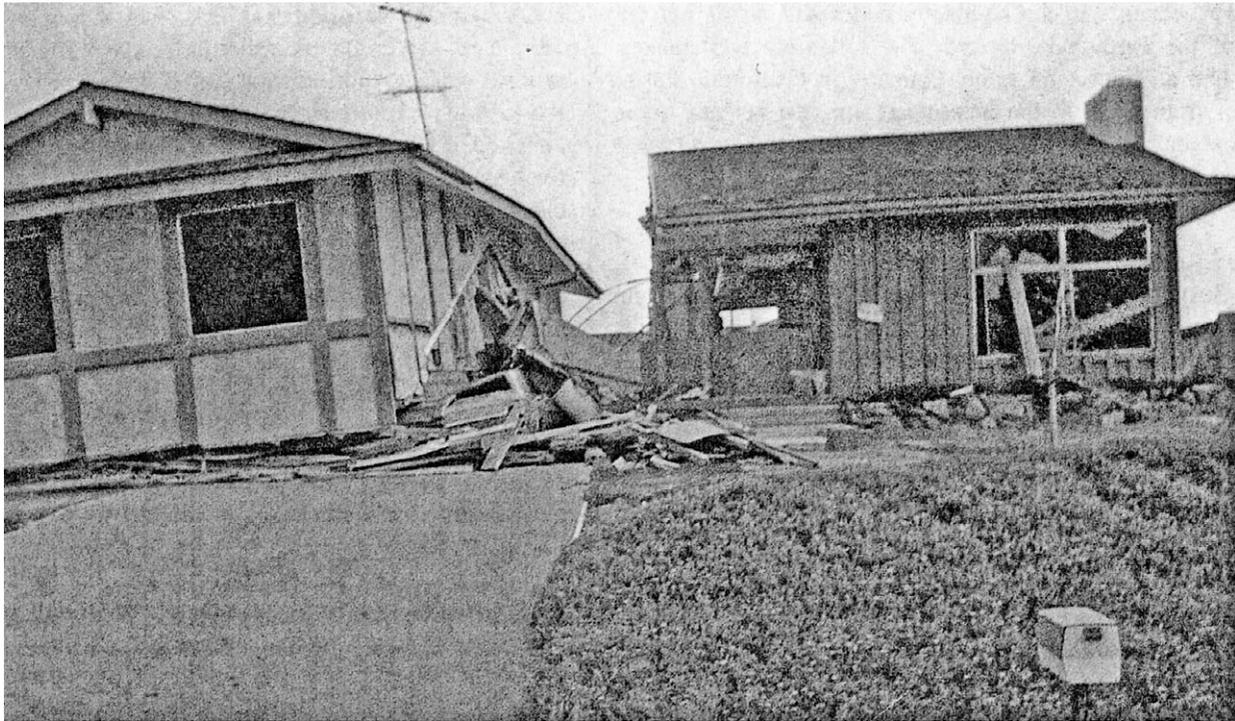
Figure 11. True split-level house in Sylmar after the 1971 earthquake. The heavier bedroom collapsed into the two-car garage during the strong ground shaking.
