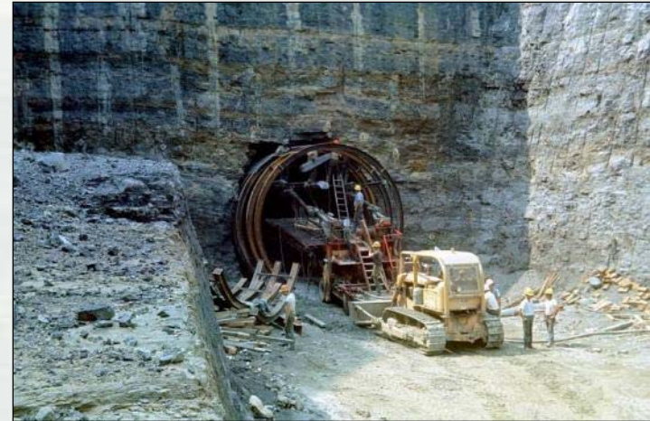
Tunnel lining frame at Outlet
