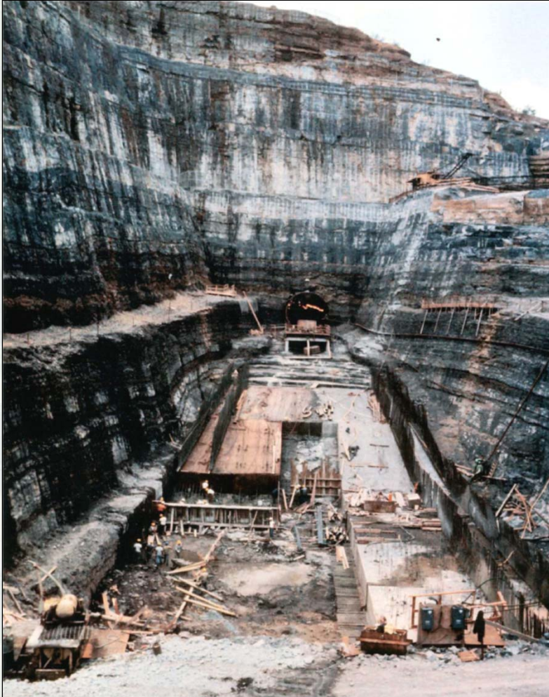
Concrete slab construction
