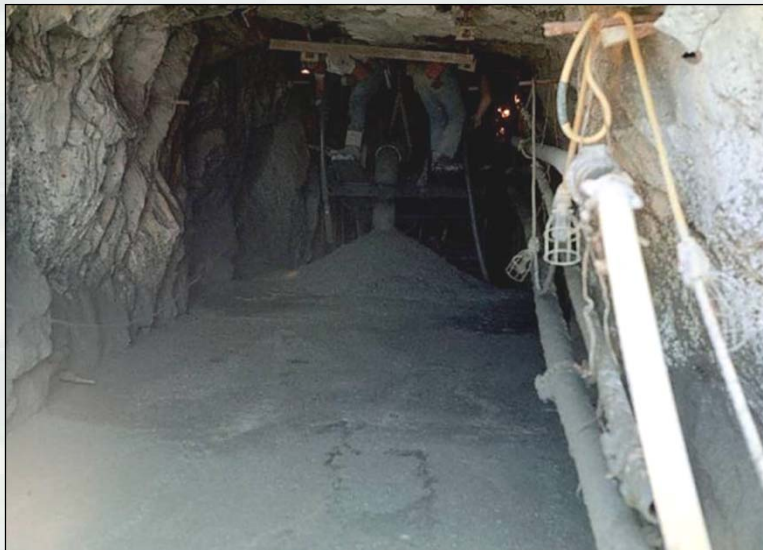
Concrete placement in Membrane
