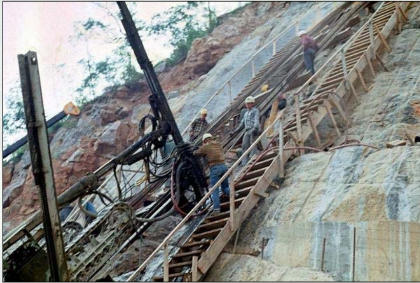
Drilling of foundation grout holes
