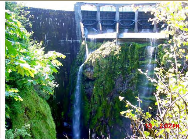
Glines Canyon Dam
