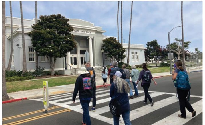
**FIGURE 5, STOP #5.** APPROACHING THE DWYER SCHOOL GYMNASIUM, ONE OF THE FEW STRUCTURES THAT SURVIVED THE 1933 M6.4 LONG BEACH EARTHQUAKE BECAUSE IT USED REINFORCED CONCRETE INSTEAD OF THE MASONRY CONSTRUCTION TYPICAL OF THE TIME.
