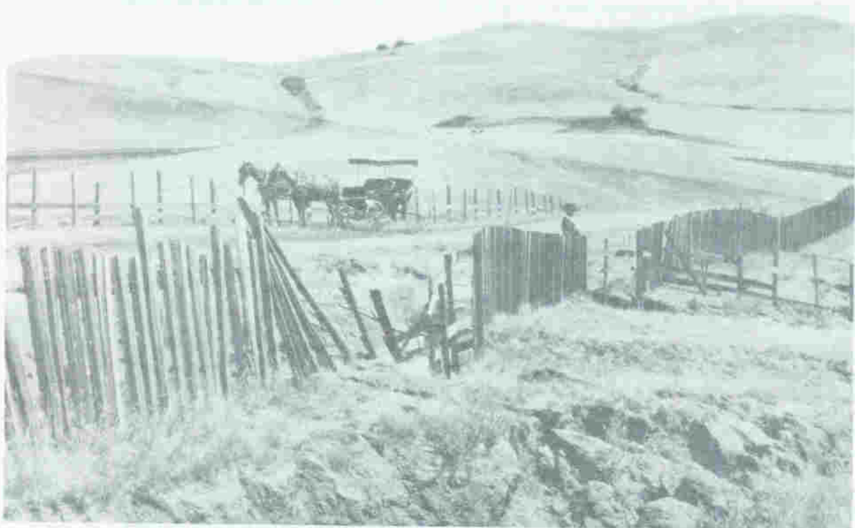
Figure 14. Offset fence at main surface break formed along the San Andreas fault near Black Mountain (now a part of Los Altos Hills) during the San Francisco earthquake of 1906.
