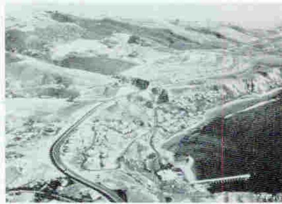
Coastwise view of the Portuguese Bend area, December 1956, showing the slide mass in left foreground. The snout of the mass emerges on the ocean bottom along the surf zone between the pier in the foreground and the white breakers in the right distance. Buckling of the pier can be seen near its shoreward end.
