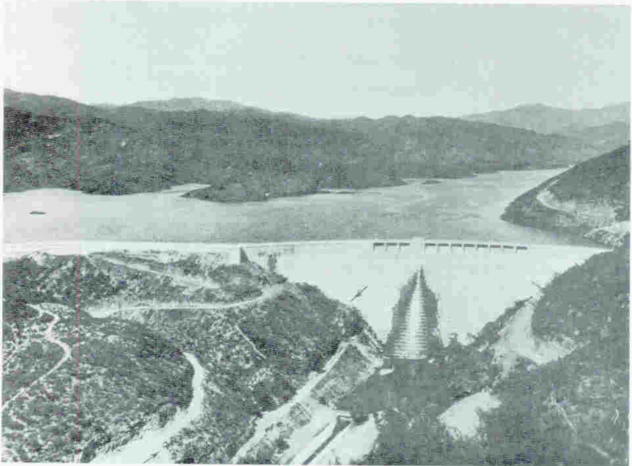
Figure 1. The St. Francis Dam, shortly before its collapse on March 12, 1928. In this upstream (northward) view, the surface trace of a major fault (between arrows) can be seen on the left-hand wall of the canyon above the lower road-bench.
