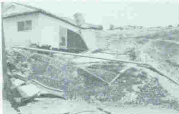
Figure 12. Acute structural distress in buildings, walls, and pavement founded on the subsiding ground shown in Figure 11.
