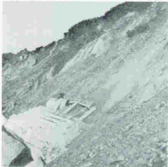
Figure 3. Broad scar of the main landslide at the easterly end of the St. Francis Dam. Here an enormous mass of bedrock (quartz-mica schist) moved downward and westward, in part against the dam, and most of it was carried away by floodwaters when the dam collapsed. The central mass of the structure remained standing, but lay out of view to the left when this photograph was taken in 1928.
