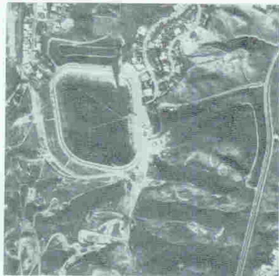
Figure 4. Vertical view of the empty Baldwin Hills Reservoir after breaching of the dam on December 14, 1963. The rapidly escaping reservoir waters created havoc in a thickly settled area of more than five square miles beyond the upper edge of this view. Pacific Air Industries photo.
