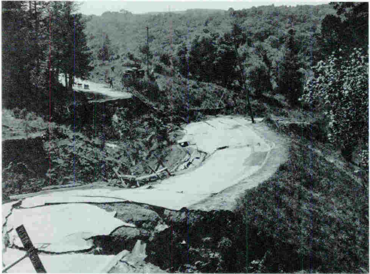
This small landslide, which occurred in Portola Valley in San Mateo County in the spring of 1967, was a reactivated portion of a much larger landslide complex that originally developed in 1890 following several years of exceptionally heavy rainfall.
