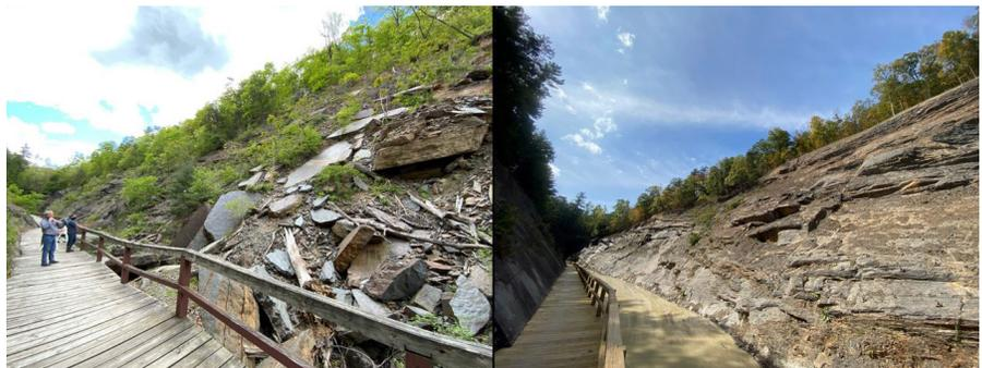
Figure 16, Paw Paw Slope Stabilization Project – As viewed looking south at the 2016 rockslide (May 2021 on left and October 2023 on right)
