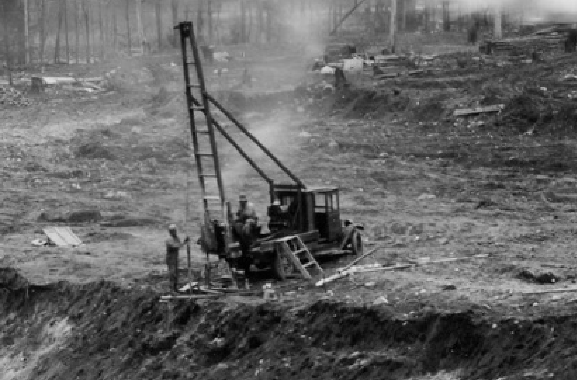
FOUNDATION EXCAVATION AND DRILLING, NOV 1929
