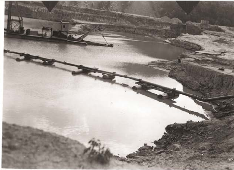
Mon. No. 20 Removal of Overburden by Dredge Photo No. 137
