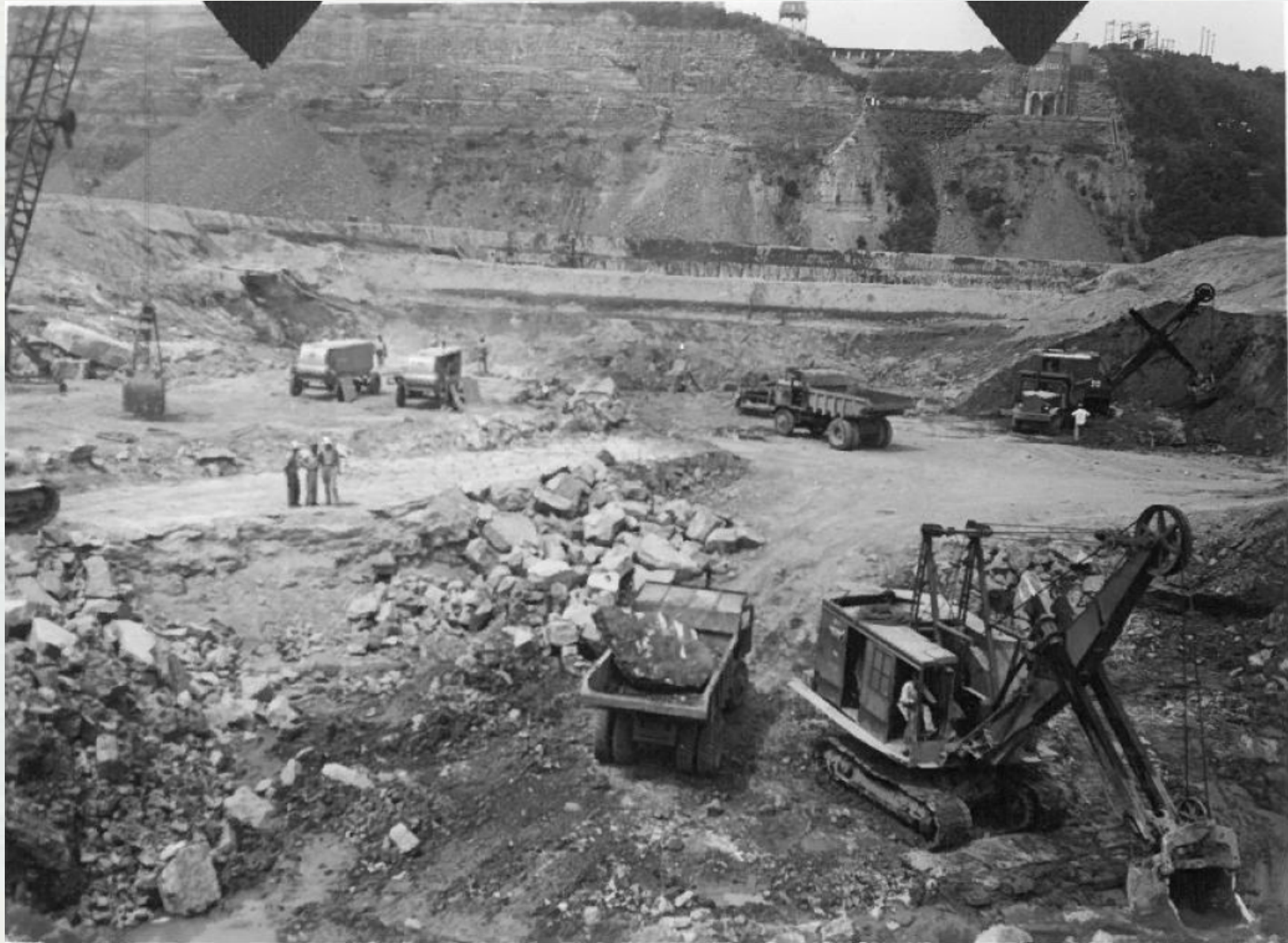
Mon.No.32 Cleaning Out Solution Channel
