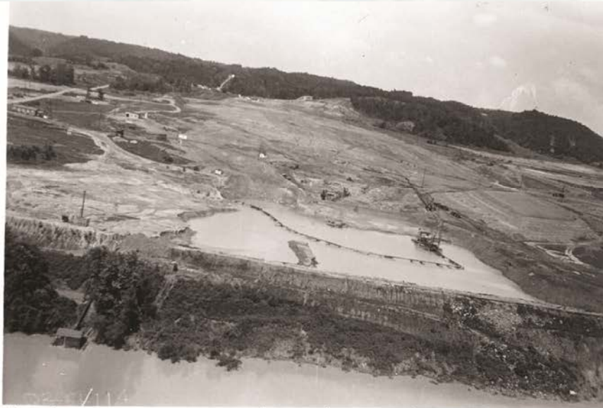
Mon. No. 20 Removal of Overburden by Dredge Photo No. 114
