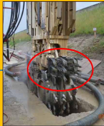
CLEANING PANEL SIDEWALLS
