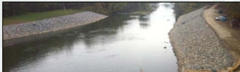
STONE SLOPE PROTECTION
