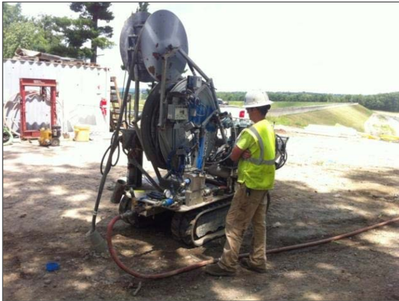
PRESSURE TESTING & GROUT CART
