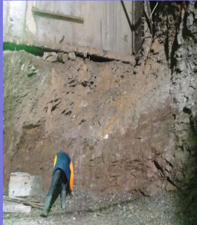
Distressing of the siltstones after excavation, under the concrete struts
