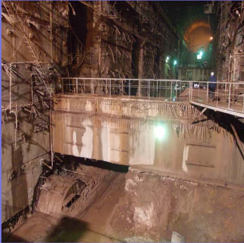
Placement of struts to face deformations
