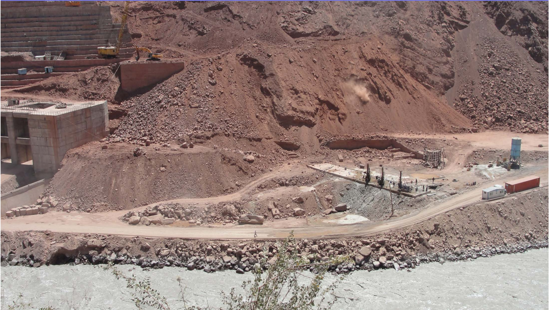
Grouting of the salt zone along the Ionakhsh fault
