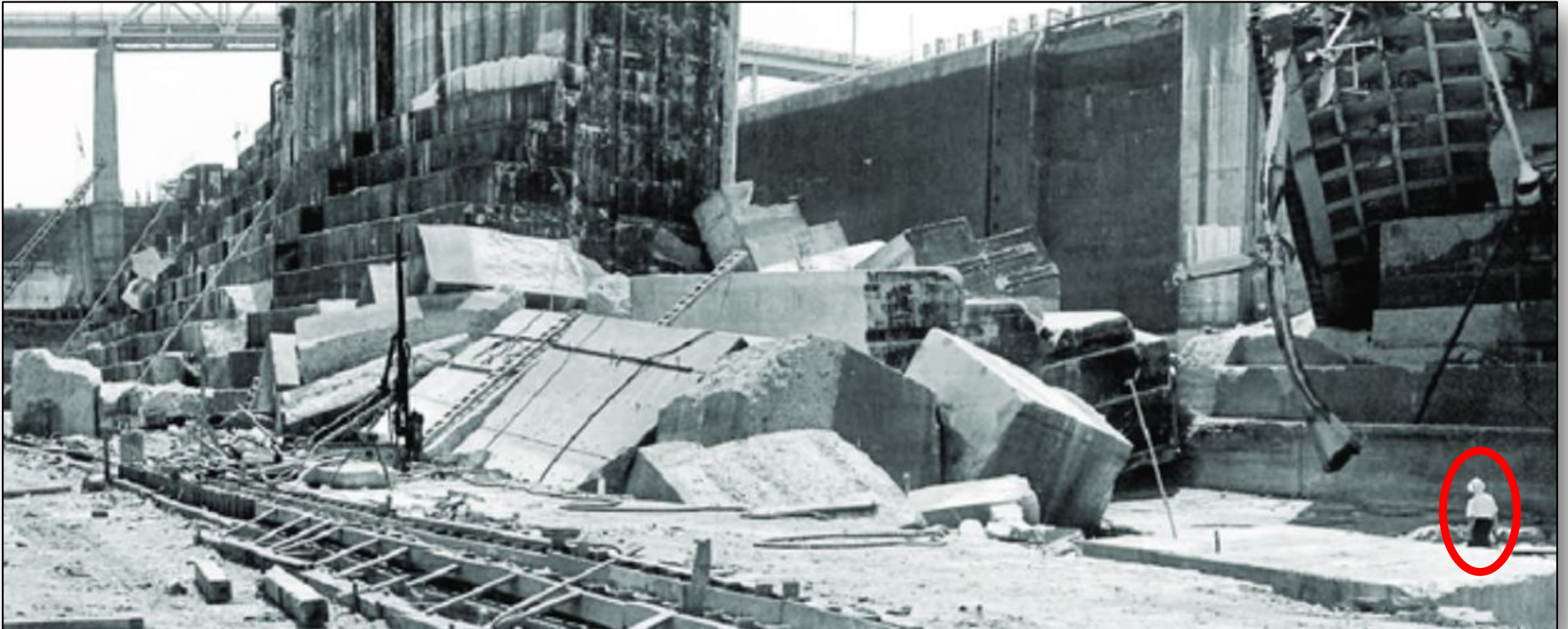
Photo Viewed from Proposed New Lock After Failure of Original Lock
