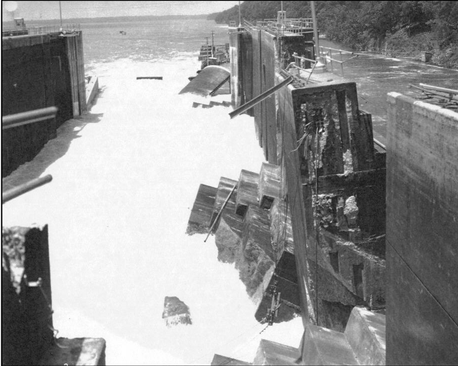
Photo Looking Downstream – After Failure
