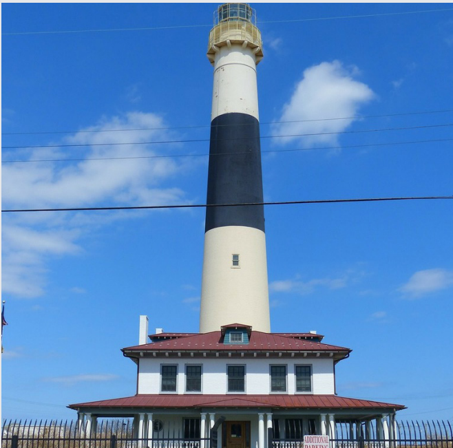
Field course 3 : Absecon Island & Brigantine Island, Atlantic County, New Jersey
