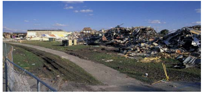
Tornado damage in Kissimmee, FL. ( Michael Collier)
